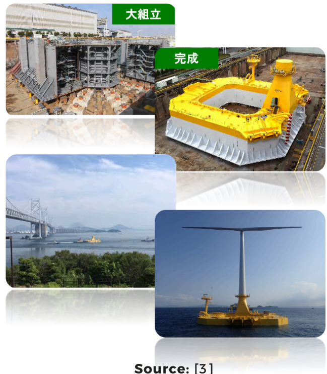
Figure 2: Phases of Hibiki FOWT life: Construction, Installation, and Operation
